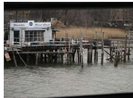
Existing Structure in Sherman Creek
